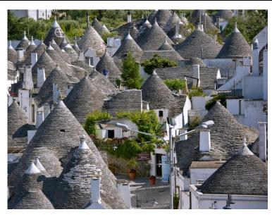
constructions are sometimes combined in a complex of communicating houses, while others are built on two levels. Most feature a grey cone-shaped roof, ending with a sphere or hemisphere shape. The interior, arranged as a single chamber, comprises niches for a fireplace, bed and furniture. The structure assures excellent indoor climate control: cool in summer and warm in winter!
