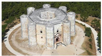
The number 8 is the principal factor in the castle's plan: 8 sides of the castle, 8 rooms on the ground floor and first floor, arranged to form an octagon, and 8 the massive octagonal towers.
